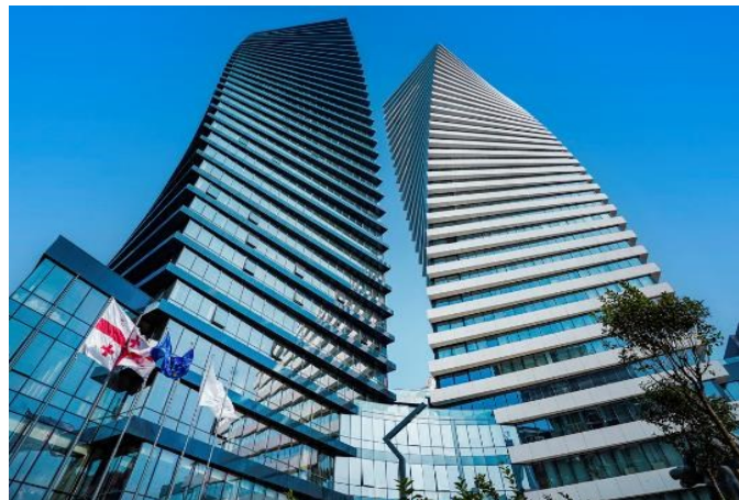
Axis Towers in Tbilisi
